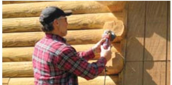
Installation of the small 1/4” backer rod is sometimes a challenge due to the design of the joint area. Here are some tips:
