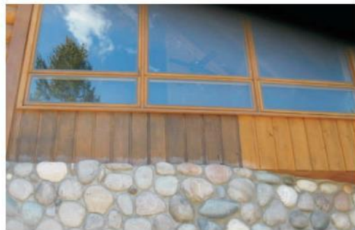
Section on left was wire brushed.
