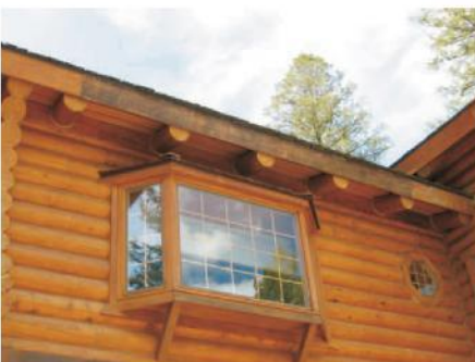
Section of fascia that was wire brushed.
