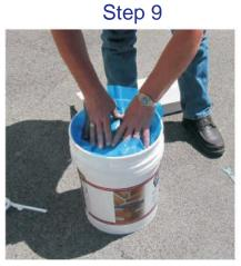
Replace plastic liner over the surface of the sealant.
