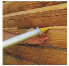
Apply sealant using the same technique as you would use with a standard caulk tube and ratchet gun.
