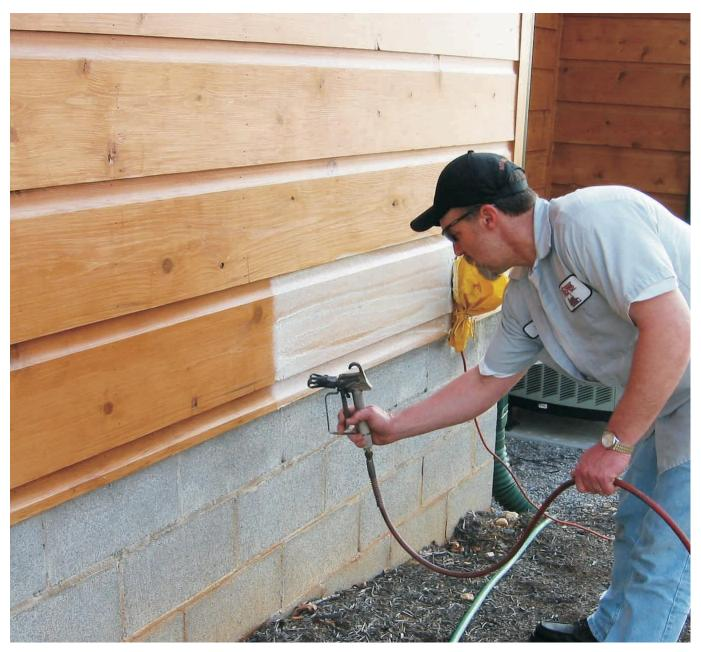
Applying S-100 Finish Remover Using a Wagner 9140S Airless Sprayer
