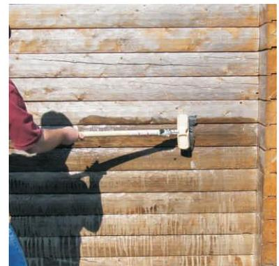
**Step 6:** Apply the Wood ReNew™ solution to the wall with a mop, broom or car wash brush. Start at the bottom of the wall and work up. Allow the solution to remain on the wall for 10 minutes.
