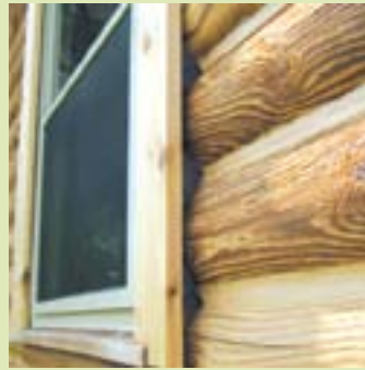
Insert Log Gap Cap™ into void between logs and frame. Leave 3/8" gap between surface of foam and edge of frame
