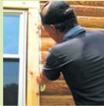
Apply masking tape to prevent sealant from smearing onto the adjacent logs
