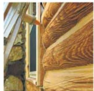
*Fill the 3/8" gap between the surface of the foam and the edge of the frame with sealant.*
