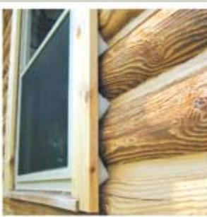
Insert foam blocks into void between logs and frame. Leave 3/8" gap between surface of foam and edge of frame.
