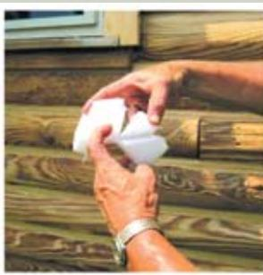
Cut triangular blocks of EPS or polyethylene foam.
