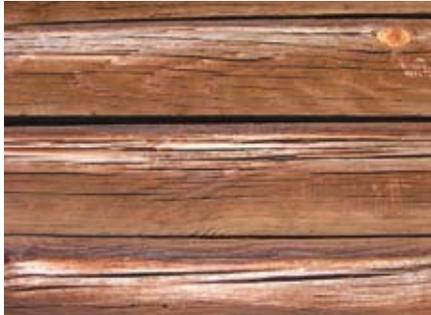
Checking and weathering of logs due to lack of maintenance.
