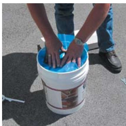
Replace the plastic liner over the surface of the sealant.
