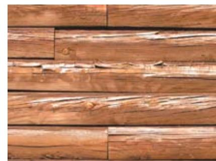
"Alligator Effect" due to weathering of unprotected surface.
