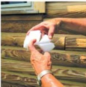
*Cut triangular blocks of EPS or polyethylene foam.*
