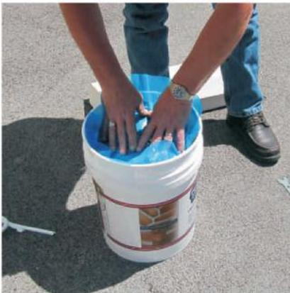
Replace plastic liner over the surface of the sealant.
