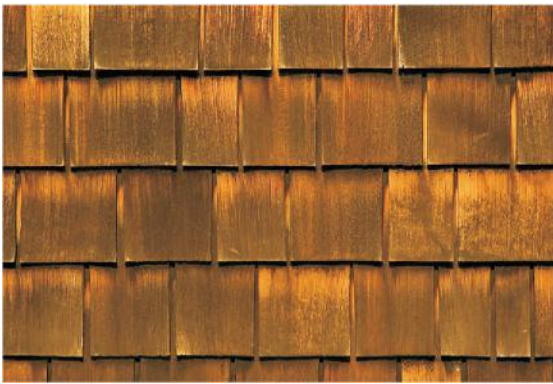
Weathered Shake Siding
