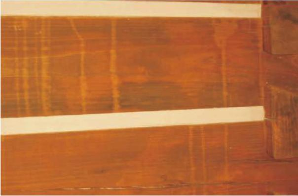
These types of discolorations usually appear within a few days. They are the result of either applying the bleach starting at the top of the wall and allowing it to run down or not adequately rinsing the bleach solution from the wall. As with all types of discolorations under the finish the only way to get rid of them is to remove the finish and start over again.
