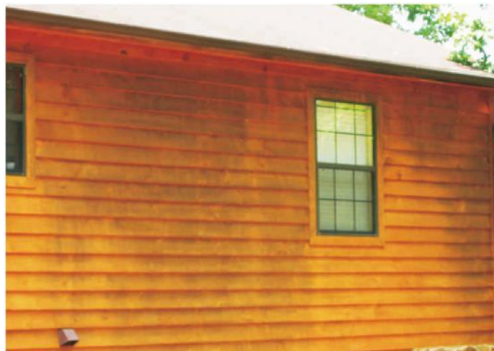
Iron tannate stains that appeared several months after the finish was applied. You can easily see where the bleach and water cleaning solution was inadequately rinsed.
