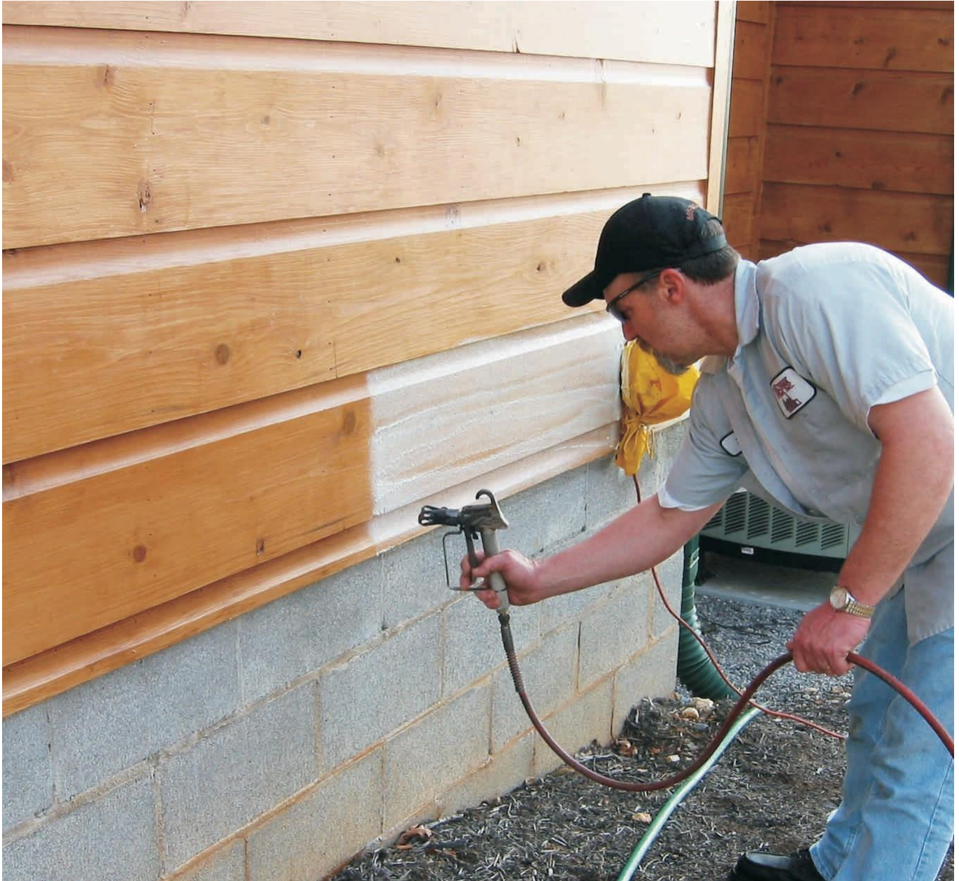
Applying S-100 Finish Remover Using a Wagner 9140S Airless Sprayer
