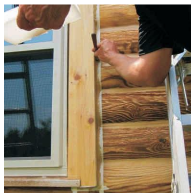
Rough tool sealant into place then lightly spray surface with water and tool smooth.
