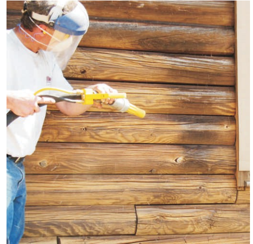
Media blasting with crushed glass
