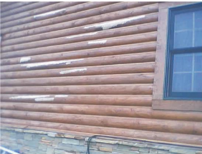
VOIDS treated with Shell-Guard RTU, M-Balm then filled with 2x4s and E-Wood.
