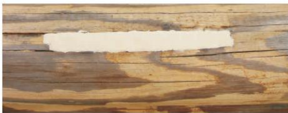
Cavity filled with E-Wood.
