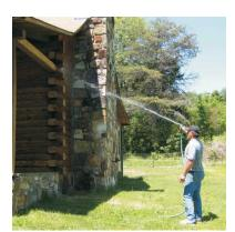
Step 3: If necessary, scrub the wall starting at the bottom and work up then rinse from the top down until you see no more
