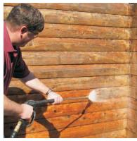
Step 7: Pressure wash starting at the bottom of the wall. Work on 2 or 3 courses of logs at a time. Hold the wand at a 30 to 45 degree angle to avoid feathering the wood.
