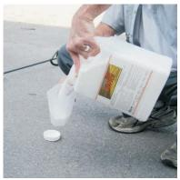
Step 2: Only measure out Step 3: enough Wood ReNew™ to add ReNew™ to a few gallons of water (0.8 contains the water. Do not mix cups per gallon) at a time. You Wood ReNew™ in a sprayer. need to use whatever you mix up within 1 to 2 hours.
