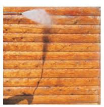
Step 8: Once the entire wall is pressure washed, rinse the wall starting at the top and work down. At this stage water volume is more important than pressure.
