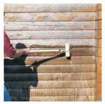
6: Wood Apply the ReNew™ solution to the wall with a mop, broom or car wash brush. Start at the bottom of the wall and work up. Allow the solution to remain on the wall for 10 minutes.
