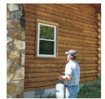
Step 1: Add 1 gallon of water to Step 2: Spray the surface with your sprayer then add the mixed Log Wash solution. approximately 2 cups of Log Start at the bottom and work up. Wash. If you add the Log Wash Allow 10 to 15 minutes contact first the sprayer will fill with time. Do not allow the surface to foam running down the wall. dry.
