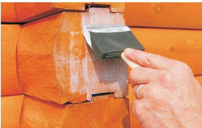
Applying Log End Seal
