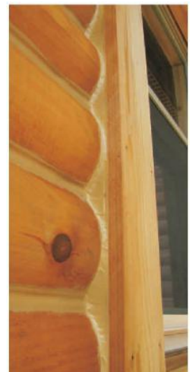
Properly sealed window trim.
