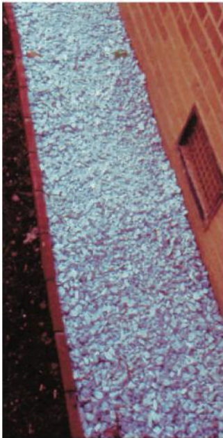
Crushed stone mulch.
