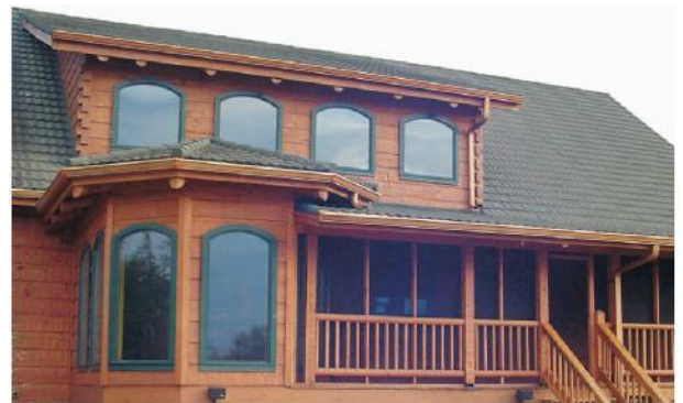
Log home properly equipped with gutters.
