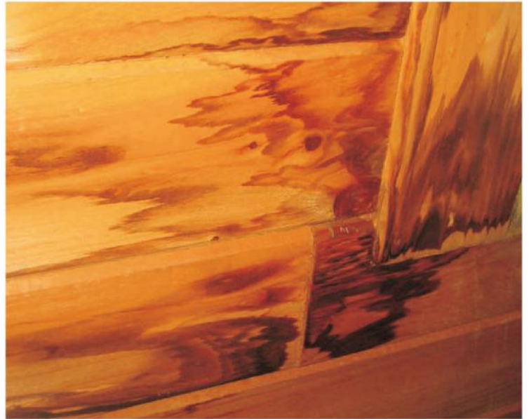
Interior Water Stains Under a Finish
