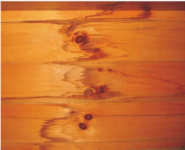
Interior Water Stains Under a Finish
