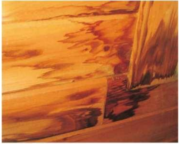
Interior Water Stains Under a Finish
