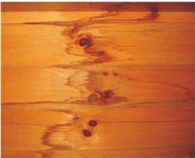
Interior Water Stains Under a Finish
