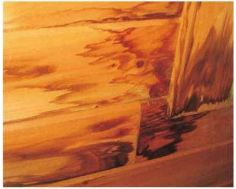
Interior Water Stains Under a Finish
