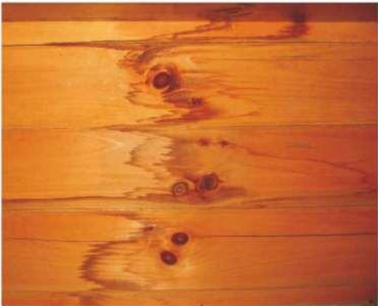
Interior Water Stains Under a Finish
