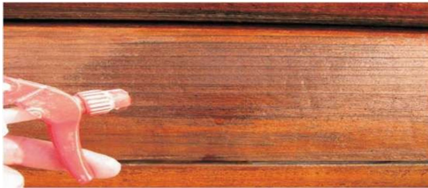
Water absorbing into the wood through a finish that is no longer water repellent
