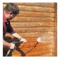
7: Pressure wash starting at the bottom of the wall. Work on 2 or 3 courses of logs at a time. Hold the wand at a 30 to 45 degree angle to avoid feathering the wood.
