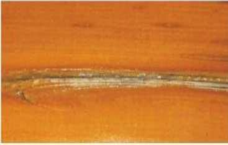
Fissure with peeling.
