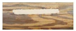
Cavity filled with E-Wood.
