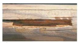
Cleaned out decayed pocket with some loose wood fibers.
