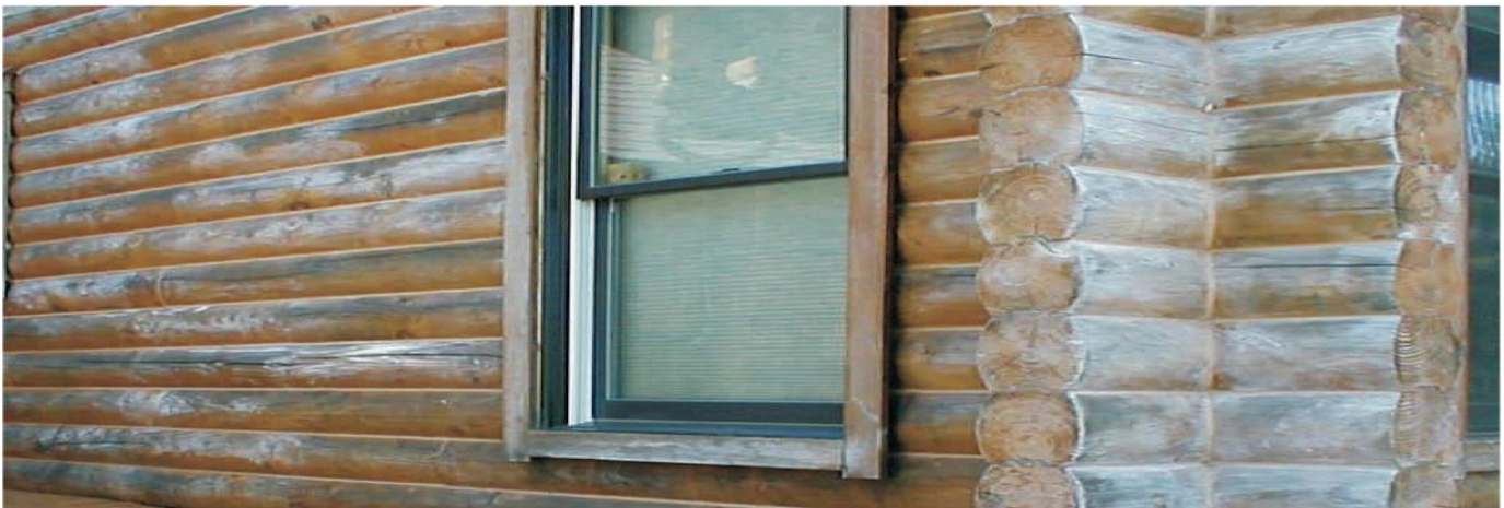
Inadequately mixed LIFELINE™ Advance Satin applied to home.
