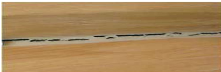
Sealant applied without a backing material to a joint between unseasoned logs.
