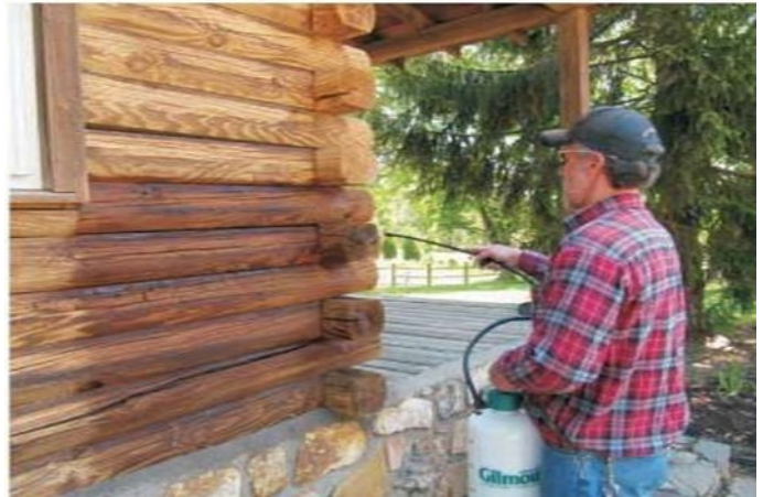
Borate solutions must be applied to bare wood.
