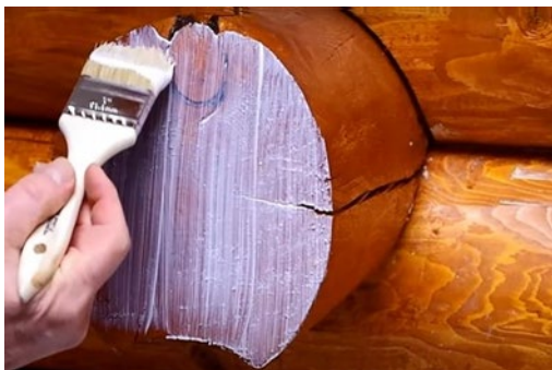
Application of Log End Seal™
