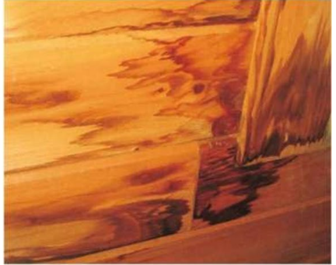
Interior Water Stains Under a Finish
