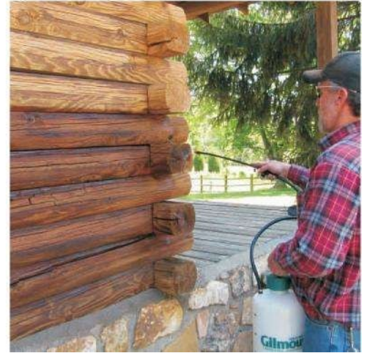
Applying a borate solution.
